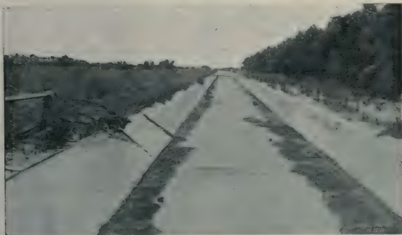
Main Channel at Mildura, 18 feet wide at bottom. (Lined with concrete.)
